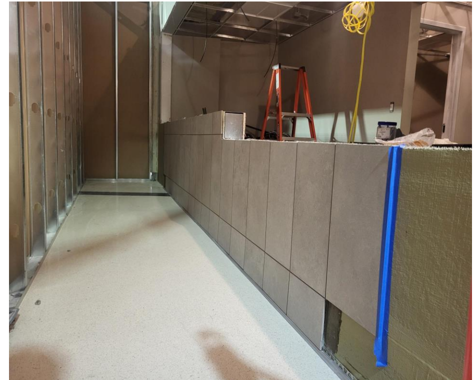
Tile wall installation
