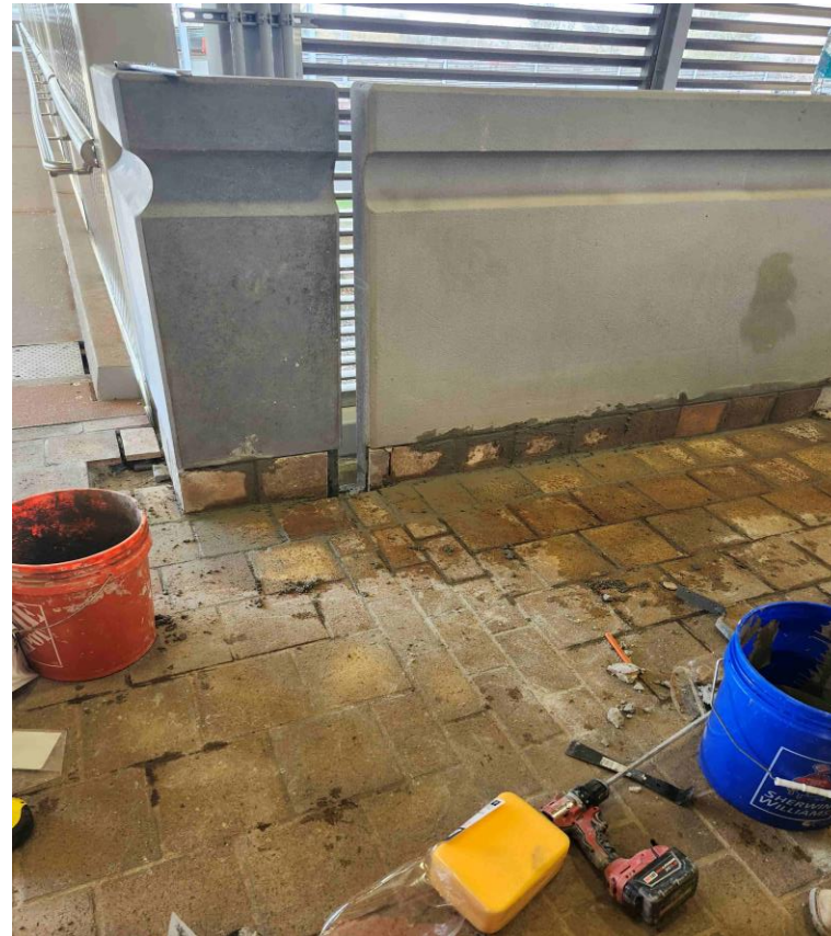
North pedestrian bridge installation
